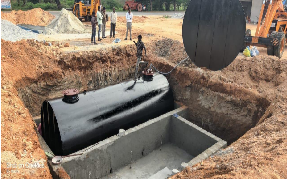
Photographs showing concrete protection wall around storage tank
